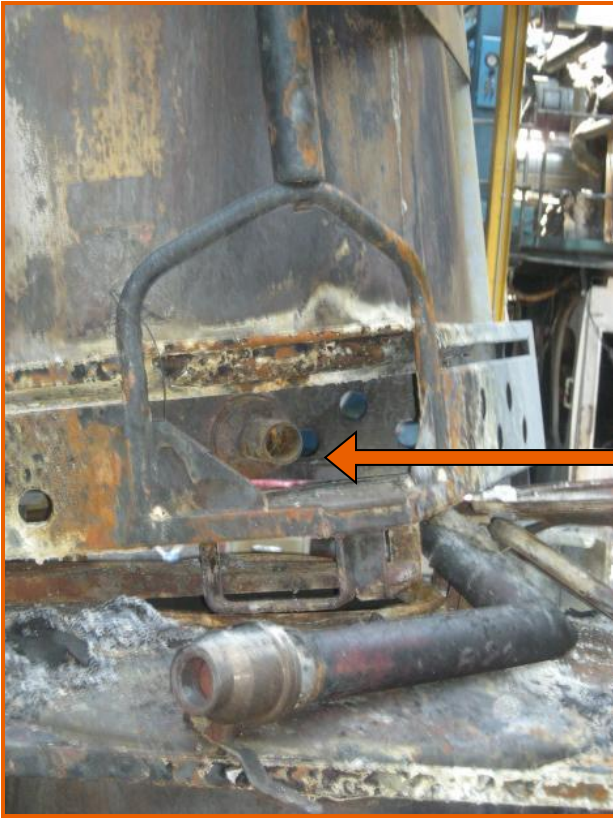
Figure 2. Tank opening without the valve
